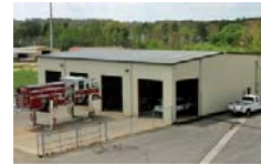
Motor Maintenance Facility
